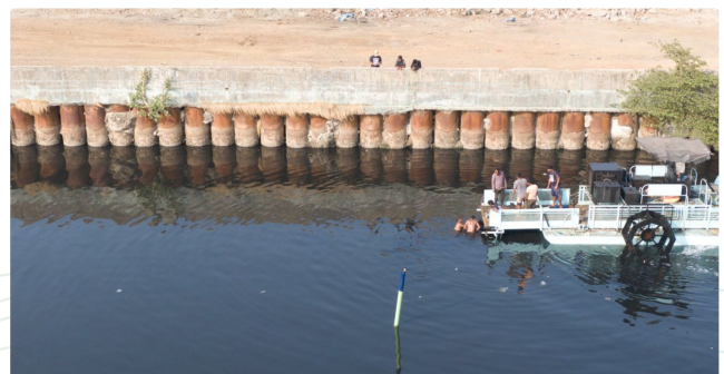
The solar-powered recovery unit, from above.
